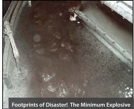
**Footprints of Disaster!** The Minimum Explosive Concentration (MEC) for PRB coal is so low, that when you see footprints immediate action should be taken to minimize the hazard.
